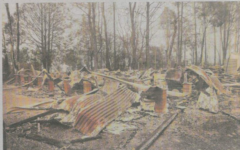
Risky business: Failure to insure against bushfire can bring disaster for families.
